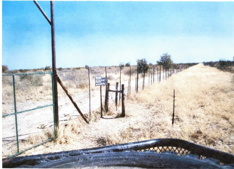
Entrance Gate & Typical Game Fencing
